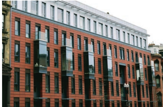
691 Massachusetts Avenue, Unit 204 - South End Nextdoor Realty Team, 617.543.4185
