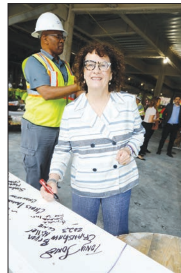
Pine Street Inn's President and Executive Director Lyndia Downie signs a 24-foot long prefabricated roof truss.
