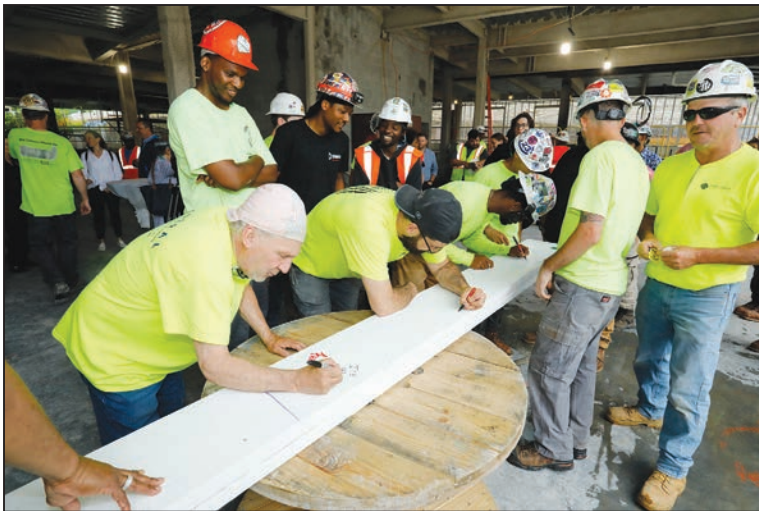
Construction workers sign a 24-foot long prefabricated roof truss during the topping off ceremony at 3368 Washington Street in Jamaica Plain.
