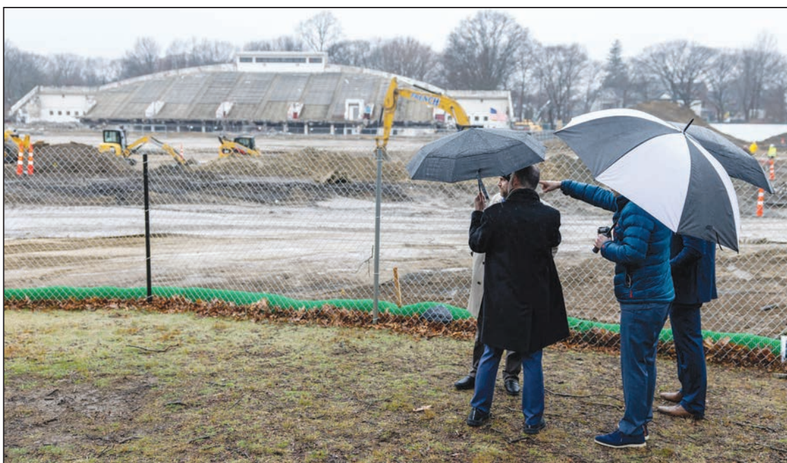
Demolition work is underway at White Stadium
