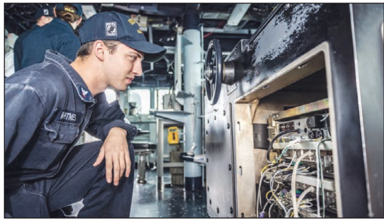
Electronics Technician 3rd Class Morgan Whitney, from Jamaica Plain, checks the connections in the ship's control console before the helm is removed on the bridge of the Arleigh Burke-class guided-missile destroyer USS Milius (DDG 69). Milius is underway conducting operations in the Indo-Pacific region while assigned to Destroyer Squadron (DESRON) 15, the Navy's largest forward-deployed DESRON and the U.S. 7th Fleet's principal surface force. (U.S. Navy photo by Mass Communication Specialist 2nd Class Taylor DiMartino)
